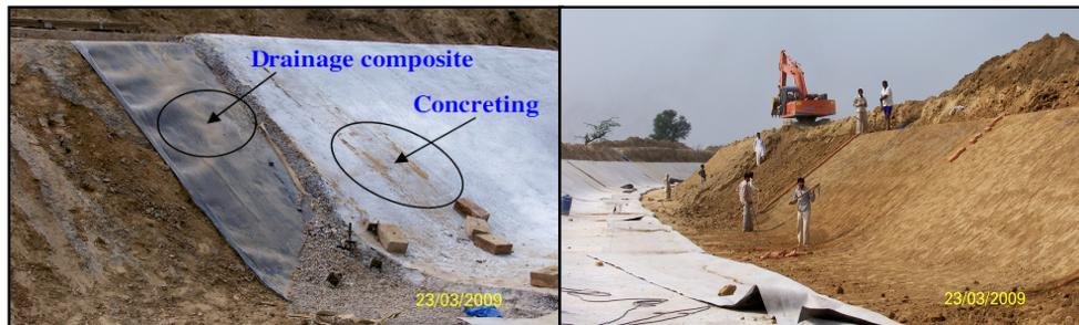
**Fig 2:** Typical Sectional details of Geosynthetics in Canal Lining
